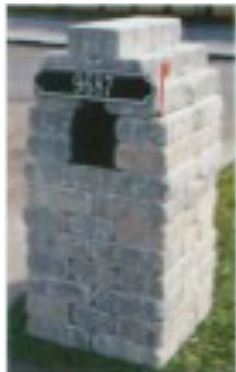
Mailbox: 67 Wall Units (4in. X 8in. X 12in.) NOTE: Rotate Pattern 90° - each layer/course
